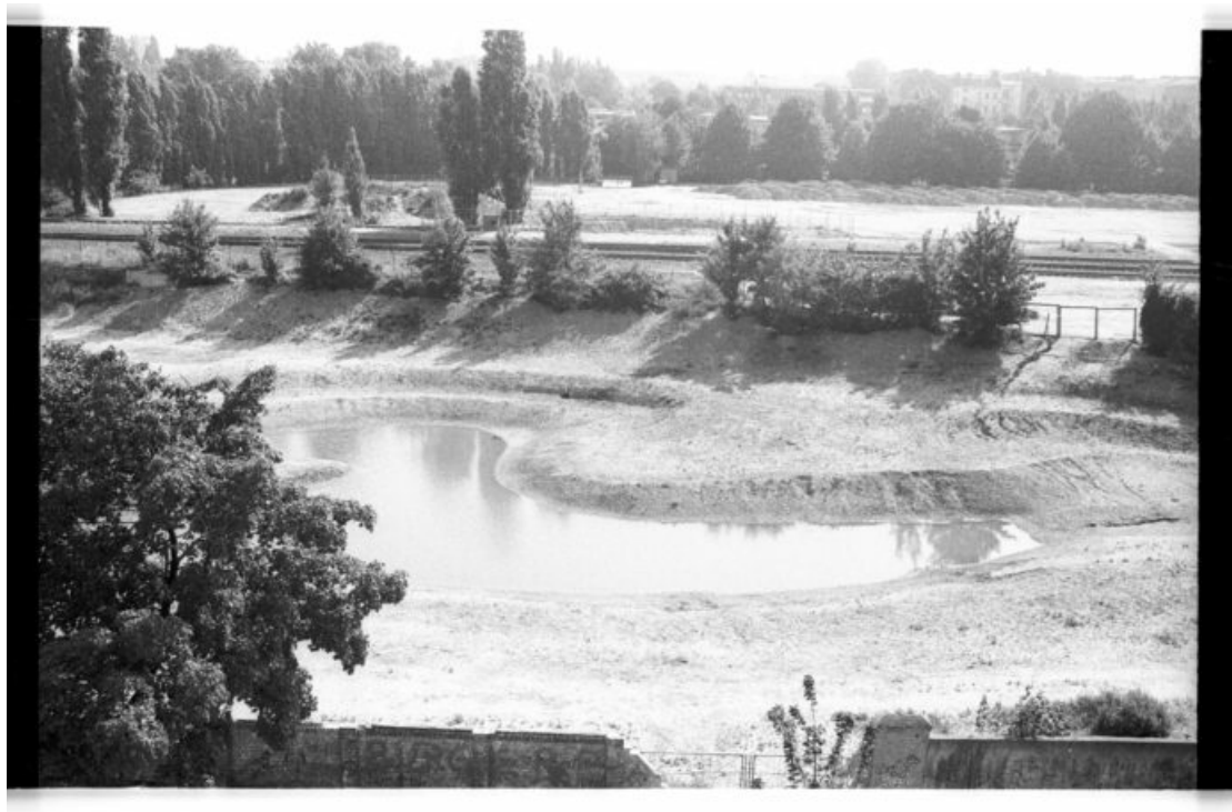
Figure 5: Photograph of the pond under construction (7 th August 1988). Source: FHXB Friedrichshain-Kreuzberg Museum, Jürgen Henschel Sammlung. Reference number: Ko3_0603_34-36.
