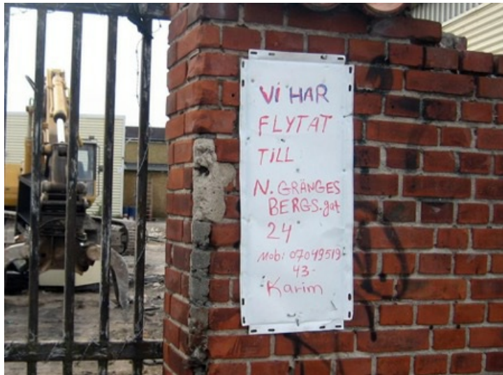
Figure 3. Östra Farmvägen 18, July 2009. The note reads (in partly inaccurate Swedish spelling): “We have moved to N.Grängesbergsgatan 24”. Source: NGBG Weblog by Oscar Ponnert.
