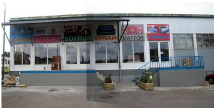
Figure 12. The exterior view of one of the wholesale stores, 2009. Source: NGBG Weblog by Oscar Ponnert
