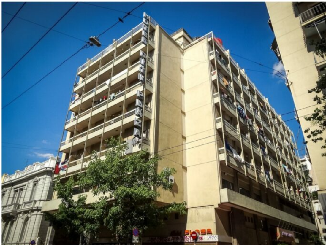
Figure 2 – The City Plaza building (March 2017). The former hotel faces the busy Acharnon street and the smaller Katrivanou street, where the only entrance is located. On the other side, the façade looks onto a quieter internal courtyard. In addition to the communal areas, there are a total of one hundred and ten rooms in the hotel, each featuring a private bathroom and a balcony. On the top floor, a large terrace overlooks the whole city, including the
