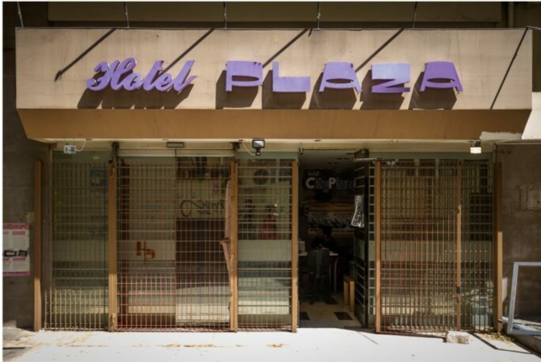
Figure 1 – The entrance to City Plaza (August 2017). The entrance door of City Plaza functioned as a threshold defining the border between an “inner” and safe space, and the “outer” and hostile urban environment. Entry to the building was only granted to residents and their guests (although the latter were not allowed to stay overnight). Immediately in front of the main door was the “security” table with activists who were in charge of checking-in people 24 hours a day in order to guarantee the safety of the hotel’s residents. It was also the task of the “security shift” to register the requests of the dozens of migrants who came to City Plaza every day with the hope of finding a place to stay.
