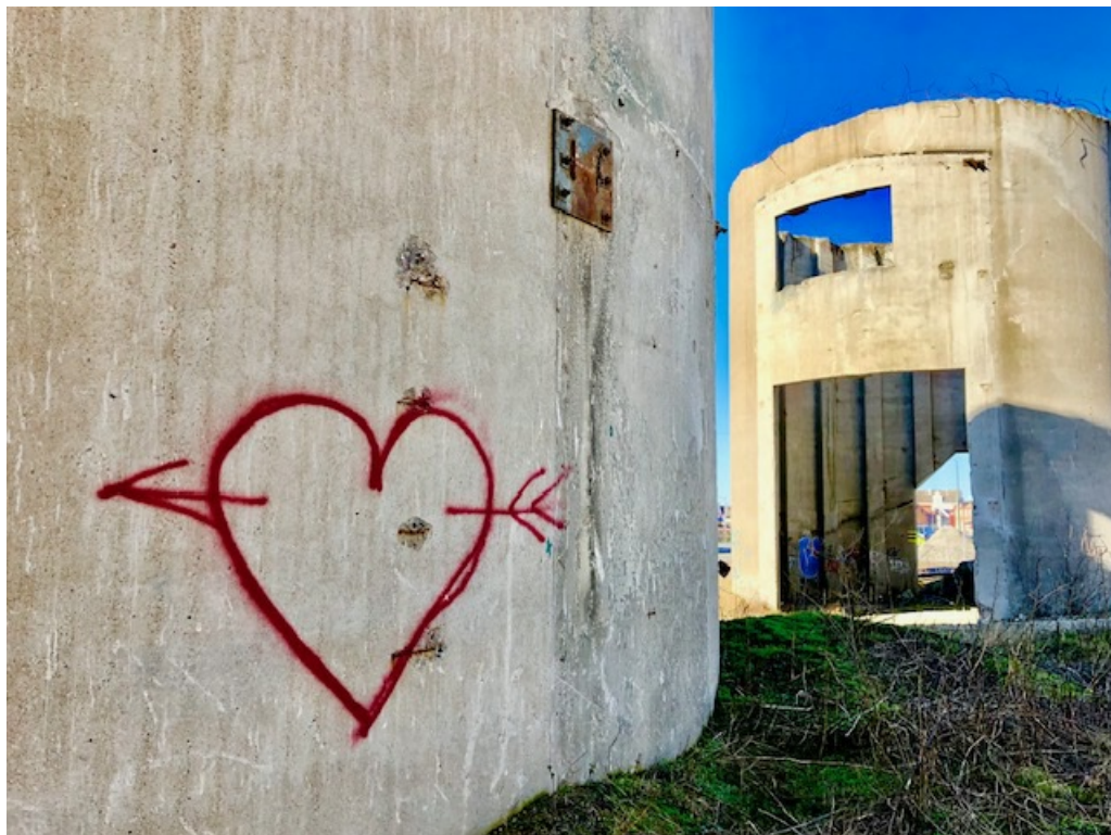
Limhamns Sjöstad, Malmö 2023. An old landmark in the industrial part of Limhamn. The silos are planned to be taken down and replaced by a high-rise building. In the meantime, they seem to be used by the local youth. How do they feel about the planned development?
