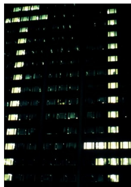
Highrise Wallpaper by Jeanelle Hurst, Qld Health Building, Outdoor Art Drive-In 1986
