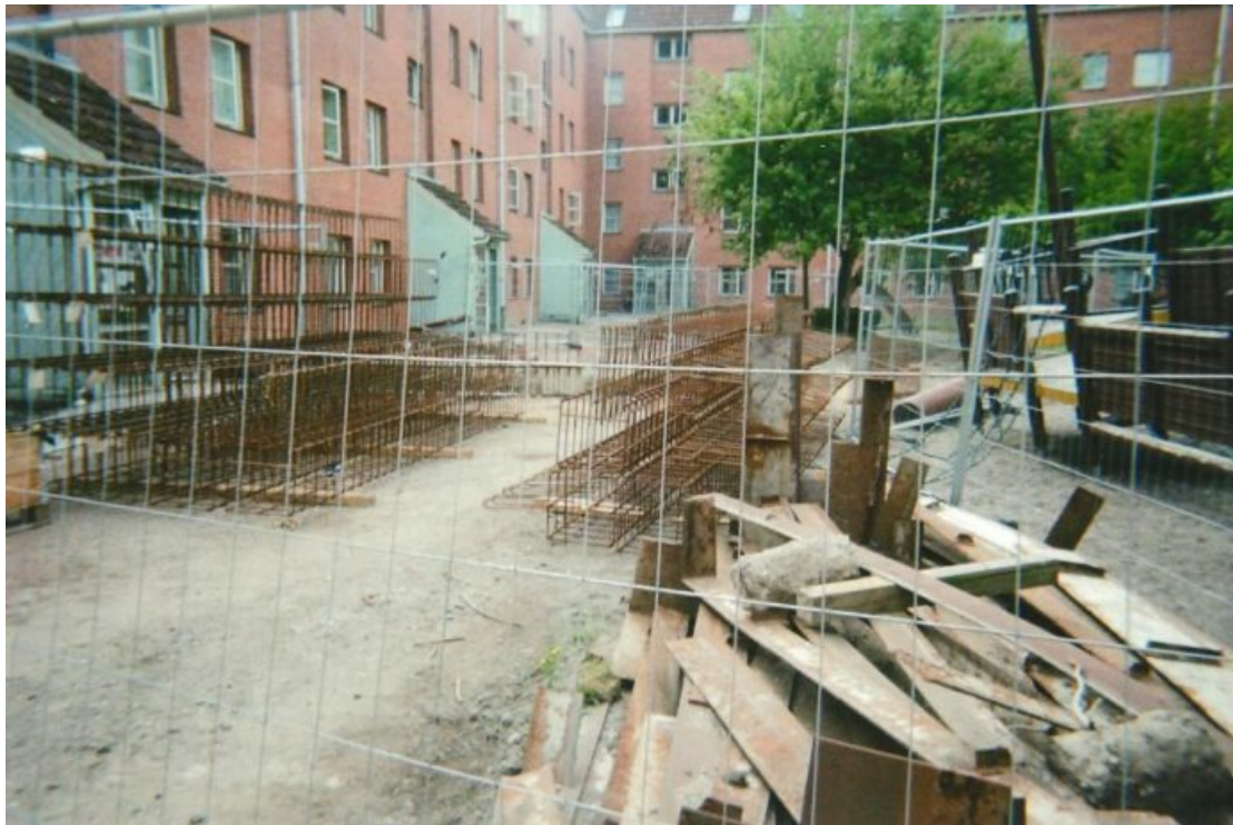
Figure 5- Piles of construction material between the entrances and the playground in yard 2, Mjølnerparken. Malika said: "There used to be a bench there, and me and my friends, we loved that bench, because it was in the shadow side. [...] I am not in Mjølnerparken that much anymore [...] because they have removed almost all the benches [...] and it is very difficult to get around, so you just want to go away. That's easiest."
