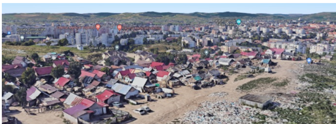
Figure 3. Slum build-up on the side of Valea Rece street (closest to viewer). Source: Google Earth Pro.
