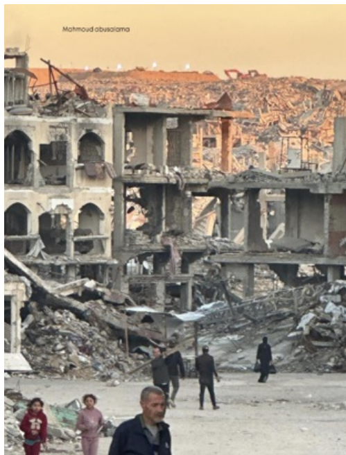
Figure 7. This image reveals the destruction of Jabalya Refugee Camp and the surrounding urban areas. Source: Mahmoud Abu Salama.
