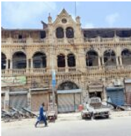
Example of a stone building 'Seth Goverdandas M. Mohatta Building' exhibiting a native and European style hybrid. Source: Author.
