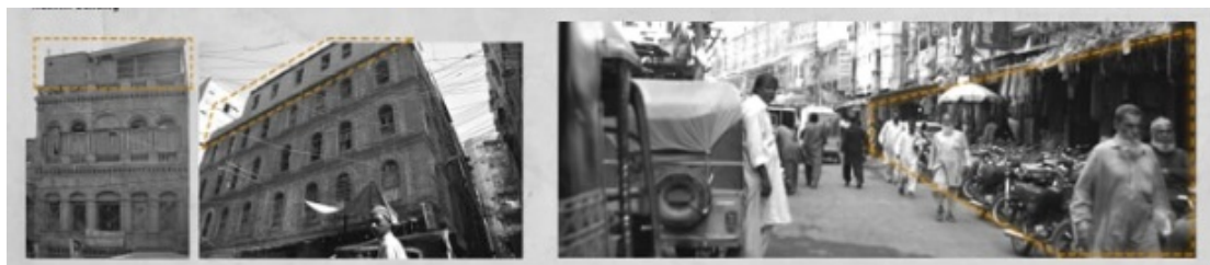
Figure IV: Images showing both horizontal and vertical based encroachments in the area. Source: Sikander et al., 2024.
