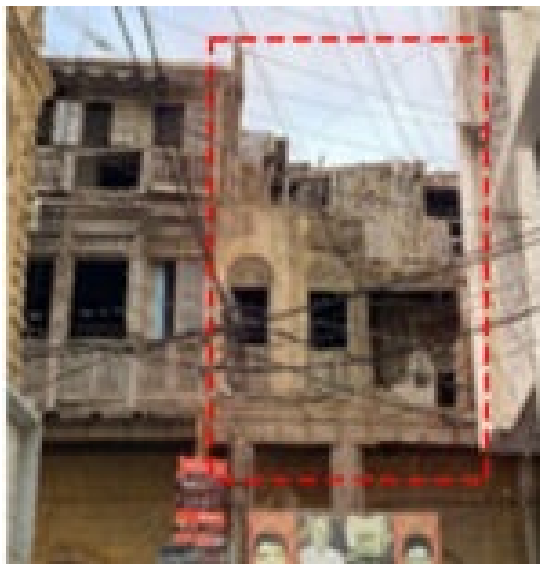
Picture of a residential building showing adobe construction. Source: Author.
